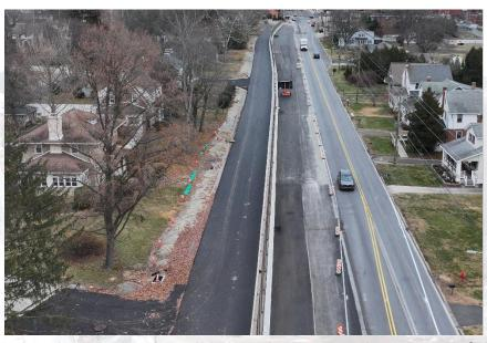
Over the winter months, the contractor will begin the Stage 2 demolition of the old bridge near McDonalds, followed by the construction of the footings and abutment walls for the new bridge. In the spring, the contractor will compete the remaining asphalt paving on the southbound side of the roadway near Township Line Road, along with the construction of a new bioretention basin and new drainage on the northbound side of the roadway.
