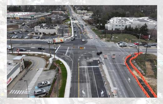
The contractor also completed the roadway reconstruction and asphalt binder course paving of Germantown Pike, to the west of U.S. 202.
