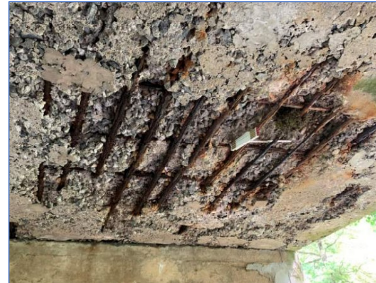
Far Right Quadrant Exposed Bars, Looking East
