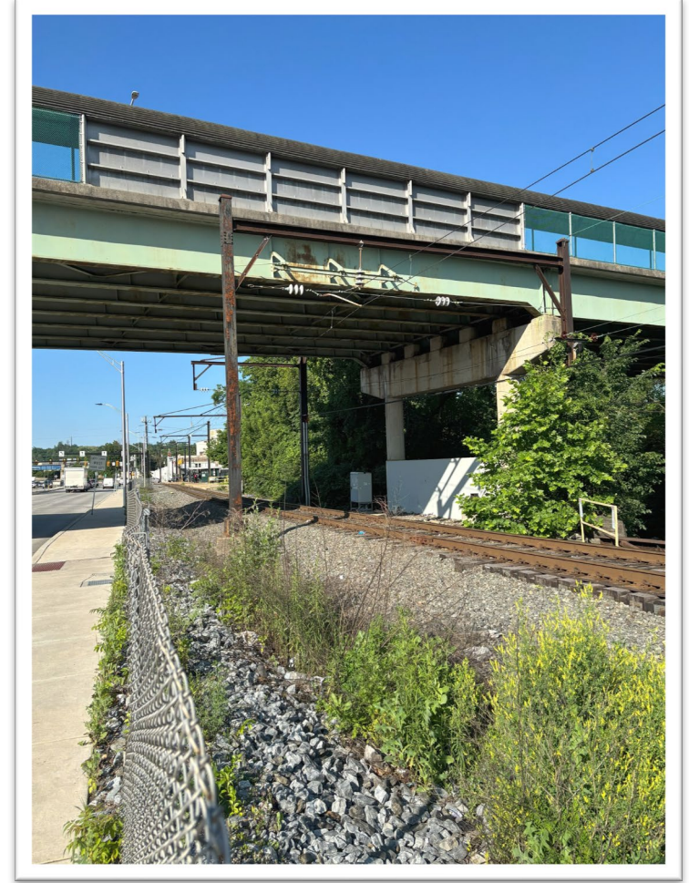
The existing vertical clearance above SEPTA railroad tracks doesn't meet current PennDOT or SEPTA requirements.
