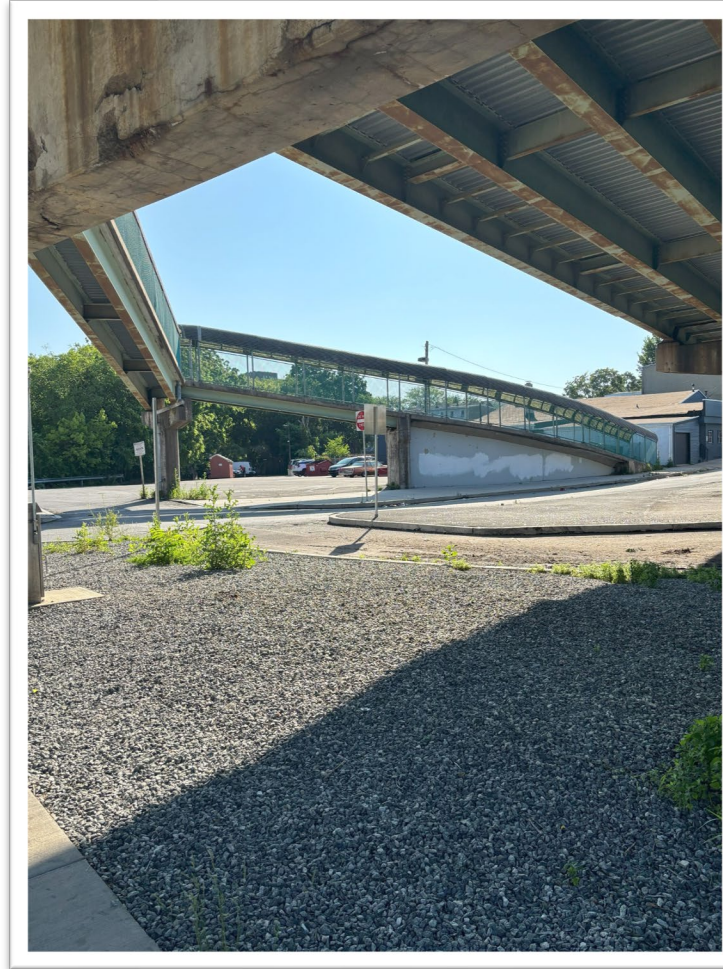
The existing pedestrian bridge ramp from the Airy Street Bridge to Markley St. doesn't meet current (ADA) standards.
