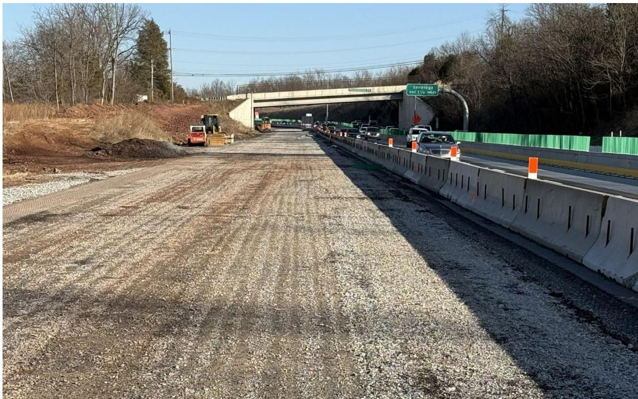
Last fall, crews removed the existing westbound asphalt (see *above*), started concrete pavement removal, and began demolition of the westbound sections of the bridges carrying U.S. 422 over Porter Road and Sanatoga Road/Sanatoga Creek (see *below*).
