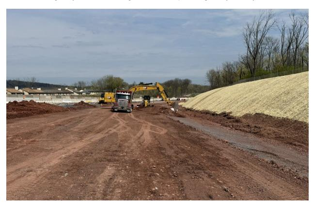
Over the winter, PennDOT's contractor made significant progress excavating and grading the eastbound side of U.S. 422 (see above) between the Norfolk Southern railroad tracks just west of Porter Road to the Sanatoga Interchange to make way for paving operations that will begin this spring and be completed in the fall.
