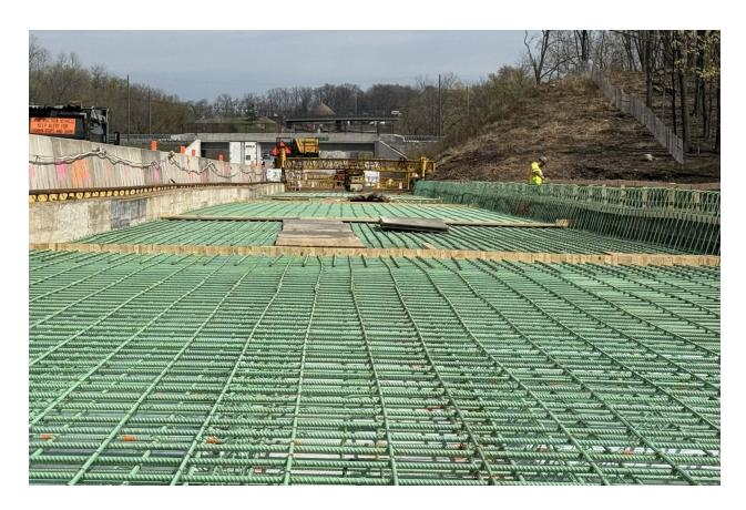
Further west, pier and abutment construction was completed last winter for the new eastbound bridge over Porter Road and Sprogels Run. Deck beams also were placed (see below), and the concrete deck will be poured this spring.
