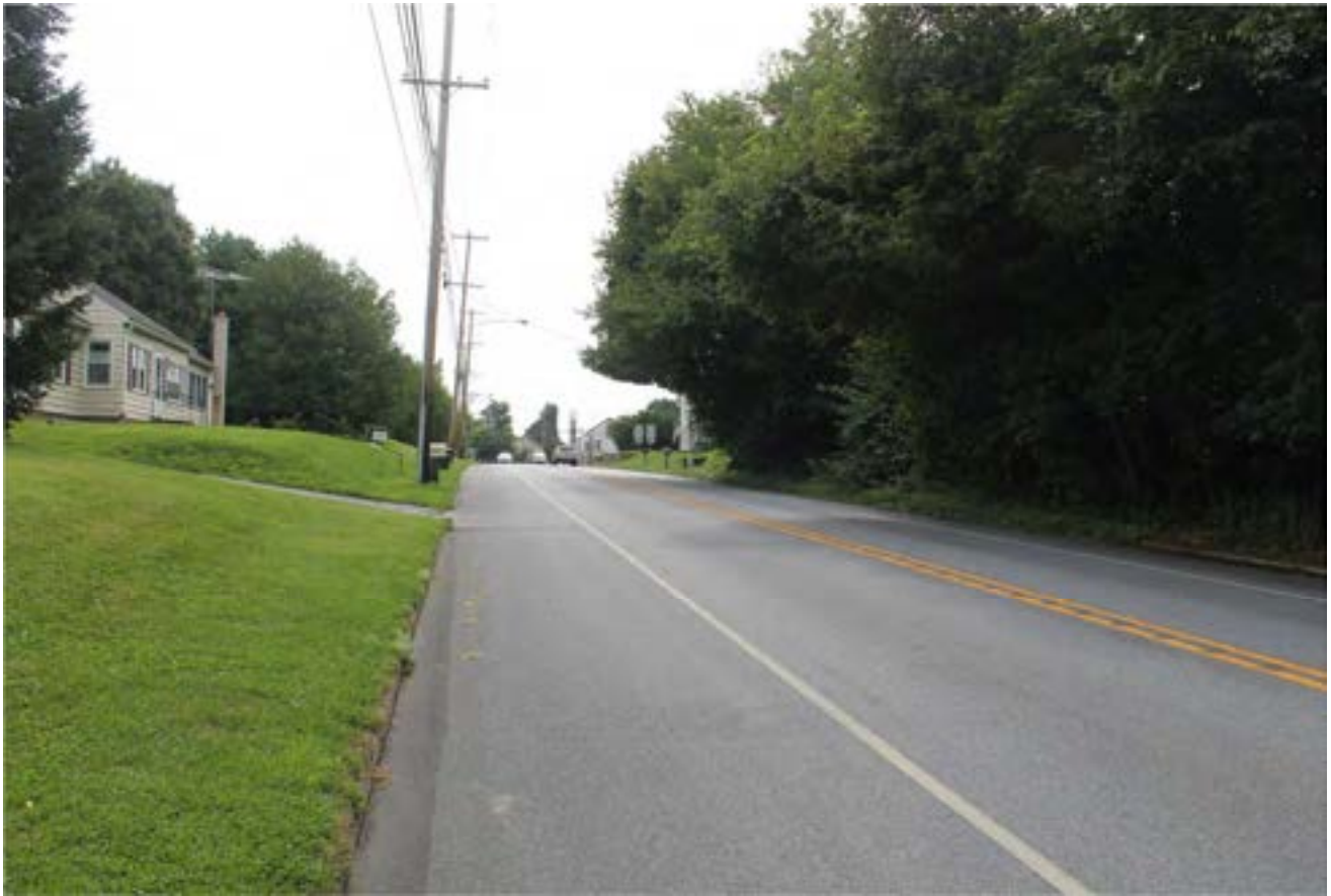
Photograph 1: View looking south along PA 41 in the village of Chatham
