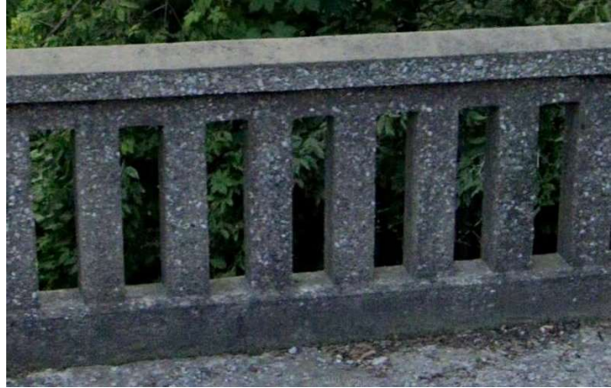
Concrete Balustrade Parapet
