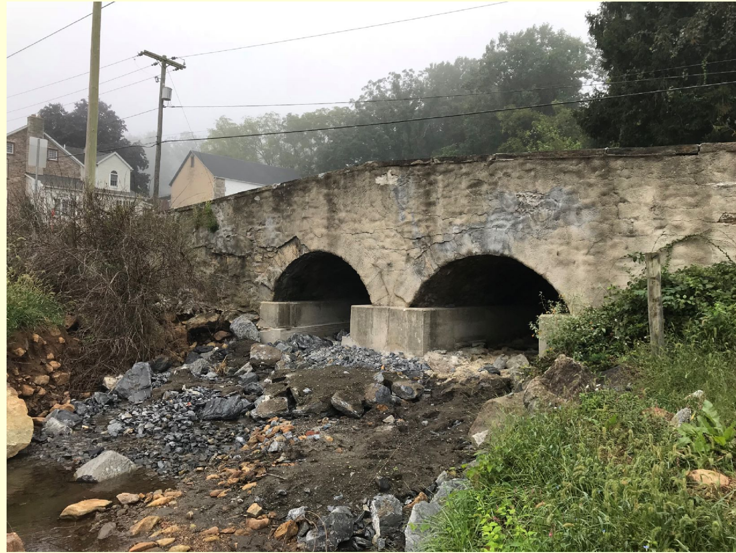
EXISTING BRIDGE ELEVATION VIEW
