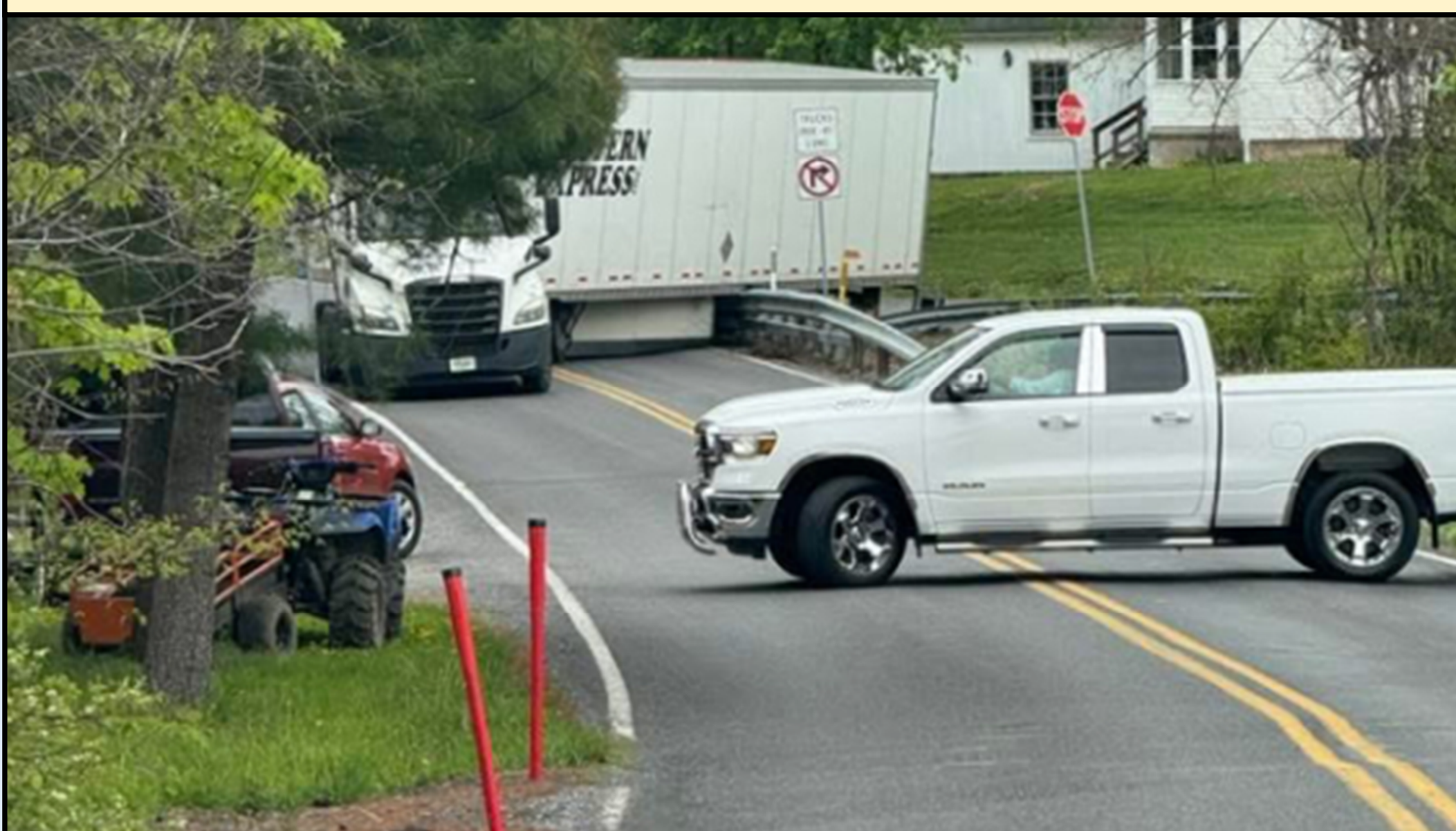
Limited turning radius at Spruce Hollow Road Intersection
