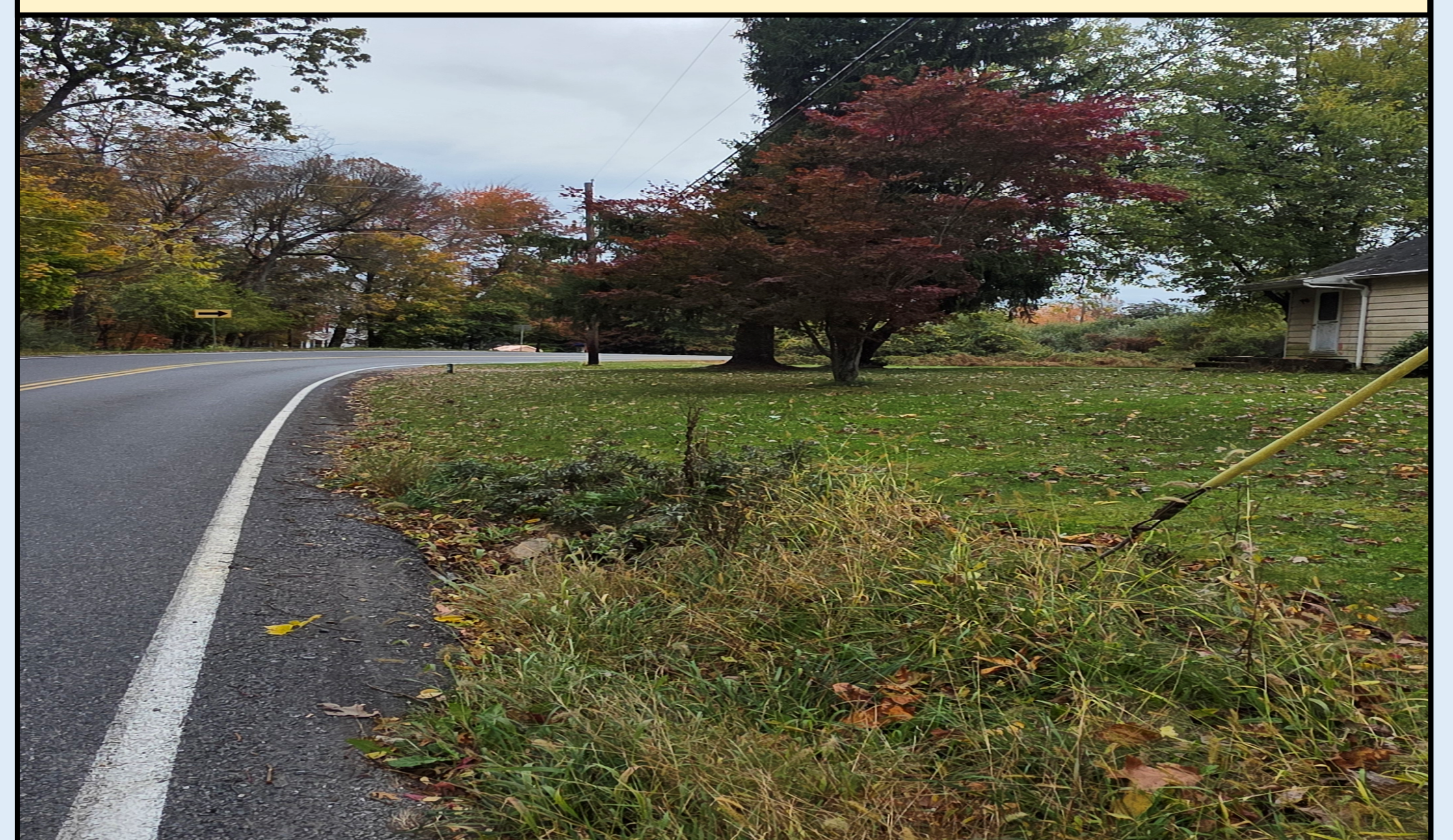
Limited sight distance through horizontal roadway curve
