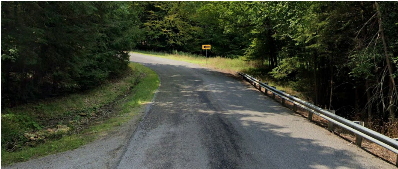
Photo 4: Looking West from Existing Structure
