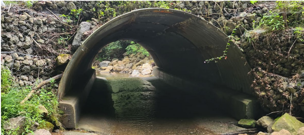
Photo 2: Upstream opening of the existing structure.
