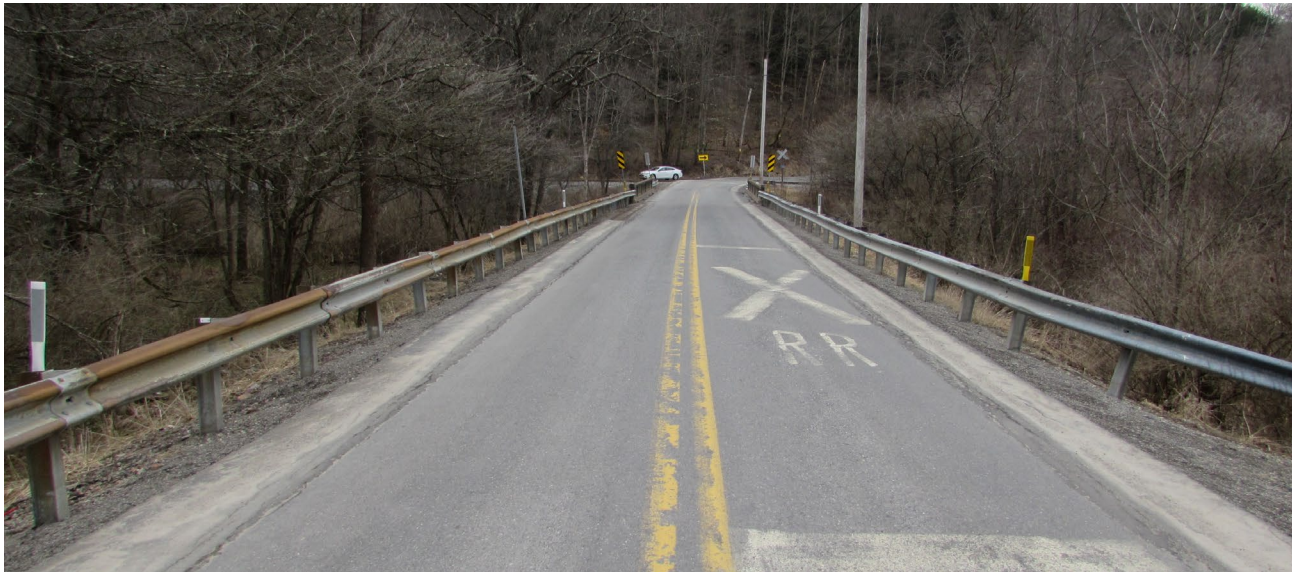
Photo 2: SR 580 looking South across structure
