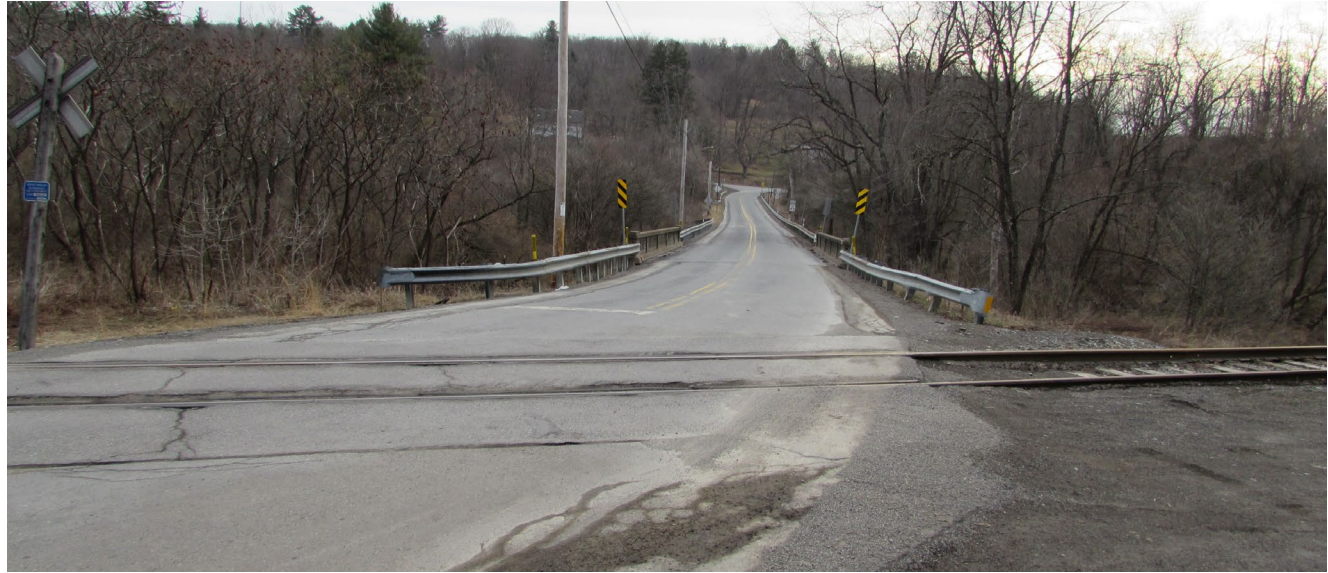
Photo 1: SR 580 looking North across structure
