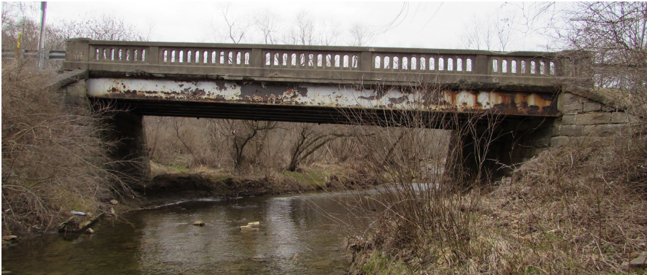
Photo 4: SR 580 looking downstream to structure
