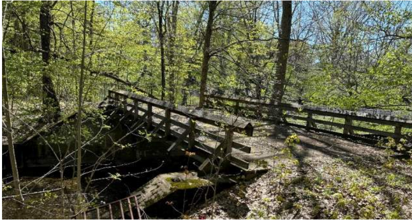
Photo 1 – Unused, existing bridge over Mill Creek connecting to Glenwood Park.
