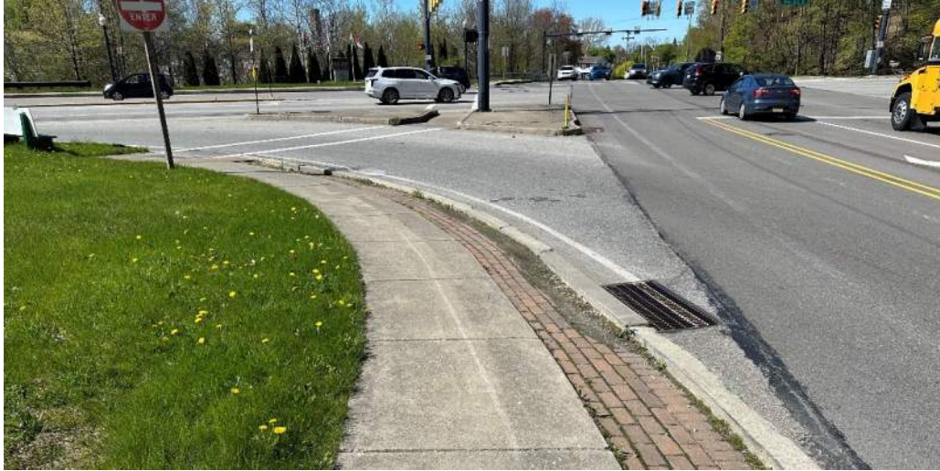
Photo 18 - Looking north at Glenwood Park Avenue (SR 505) intersection with West 38th Street (SR 4016). Pedestrian cross walk and signals.
