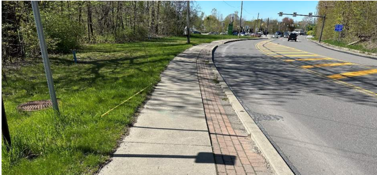
Photo 17 - Looking north along Glenwood Park Avenue (SR 505) toward West 38th Street (SR 4016), north of old 38th Street bridge.
