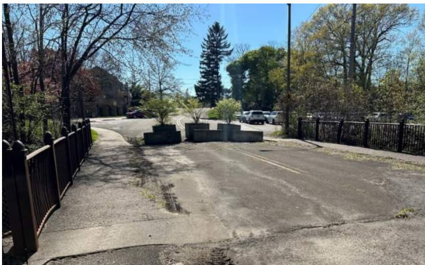
Photo 13 - Looking west across old 38th Street bridge over Mill Creek. Open to pedestrians and closed to vehicles since 2017.
