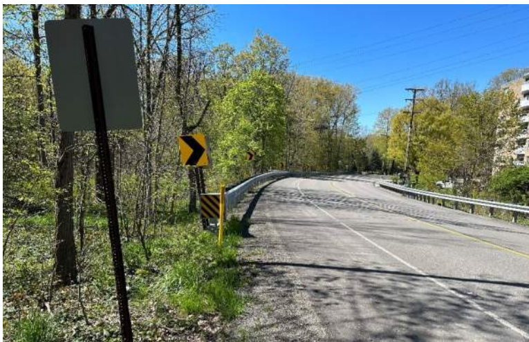
Photo 2 - Looking north along shoulder of Glenwood Park Avenue (SR 505) and bridge over Mill Creek, north of Glen Drive.
