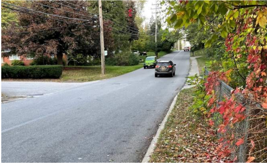
Photo 26 - Looking north on Cherry Street at culvert with chain link fence on east side.
