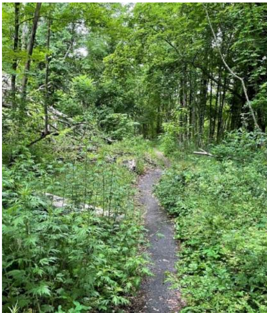
Photo 27 - Old Glenwood Park Avenue bituminous cartway with extensive overgrowth.
