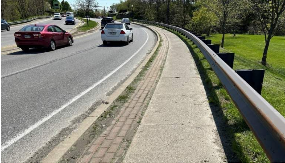
Photo 19 - Looking west along sidewalk on West 38 Street (SR 4016) , west of intersection with Glenwood Park Avenue (SR 505).
