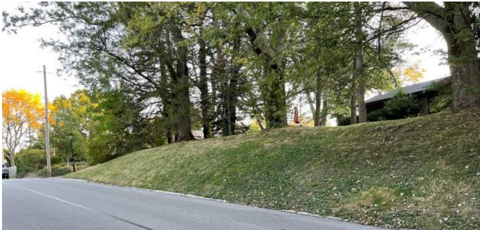
Photo 25 - Steep slope on east side of Cherry Street south of Gordon Lane.
