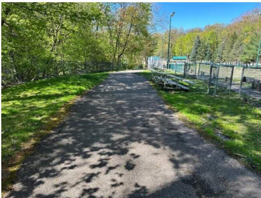
Photo 9 - Bituminous trail through Glenwood Park, looking north near horseshoe pits.
