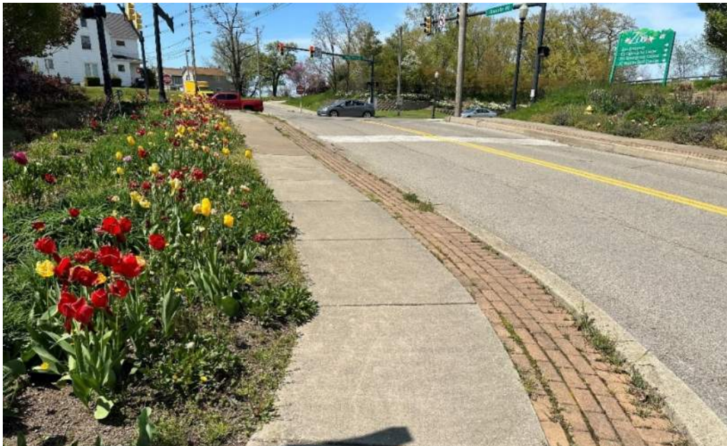
Photo 16 - Looking north along concrete sidewalk and brick pavers at the Zoo entrance drive toward West 38th Street at Shunpike Road.
