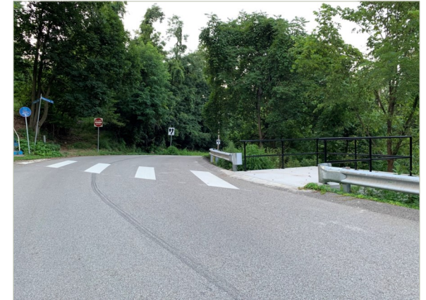
City of Pittsburgh: A Technically Infeasible Form could be useful for any future alteration request. A loading pad (“boarding and alighting area” in PROWAG terminology) provides a guiderail break for a rider to stand outside the roadway. There are no adjacent sidewalks. Stairs to a residential area are the only approach from the left, but a crosswalk has been added from the stairs to the transit stop. A required detectable warning surface (DWS), triggered by the presence of the crosswalk, is missing. (Credit: Darcy Cleaver, Pittsburgh Regional Transit)
