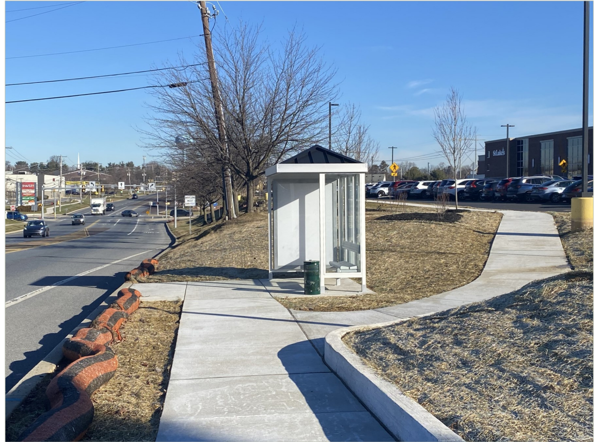
Cetronia Road at St. Luke’s West End Medical Center, South Whitehall Township, Lehigh County: This transit stop was built in conjunction with the adjacent landowner. There is a tie-in to site access. The design addresses grading changes to accommodate accessibility. Credit: Molly Wood, LANta
