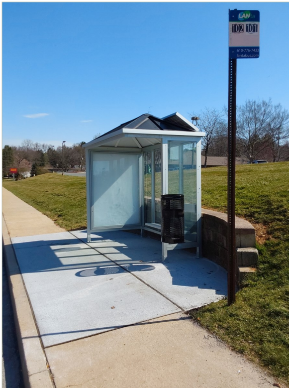
Salisbury Township, Lehigh County: Because of the grade behind the transit stop, a retaining wall was constructed and a portion of the berm removed to allow for the 5'x 8' loading pad (boarding and alighting area). Credit: Molly Wood, LANta
