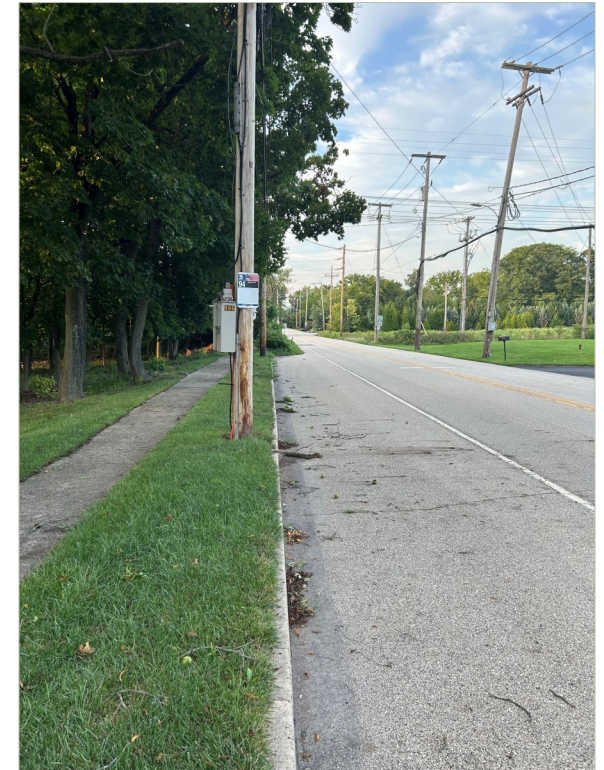
Upper Gwynedd Township, Montgomery County: This typical transit stop could accommodate alteration. The verge area (grass strip) could be traversed by a loading pad to connect the curb face with the existing sidewalk. Conversely the transit stop in the opposite direction without sidewalk or curb would require more detailed design and possibly right-of-way to alter.
