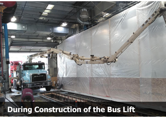
During Construction of the Bus Lift
