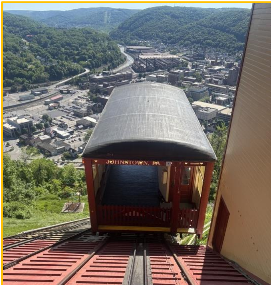
Image 10. Johnstown Inclined Plane (CamTran). May 28, 2026. This and all other photos in report taken by PennDOT SSOA.
