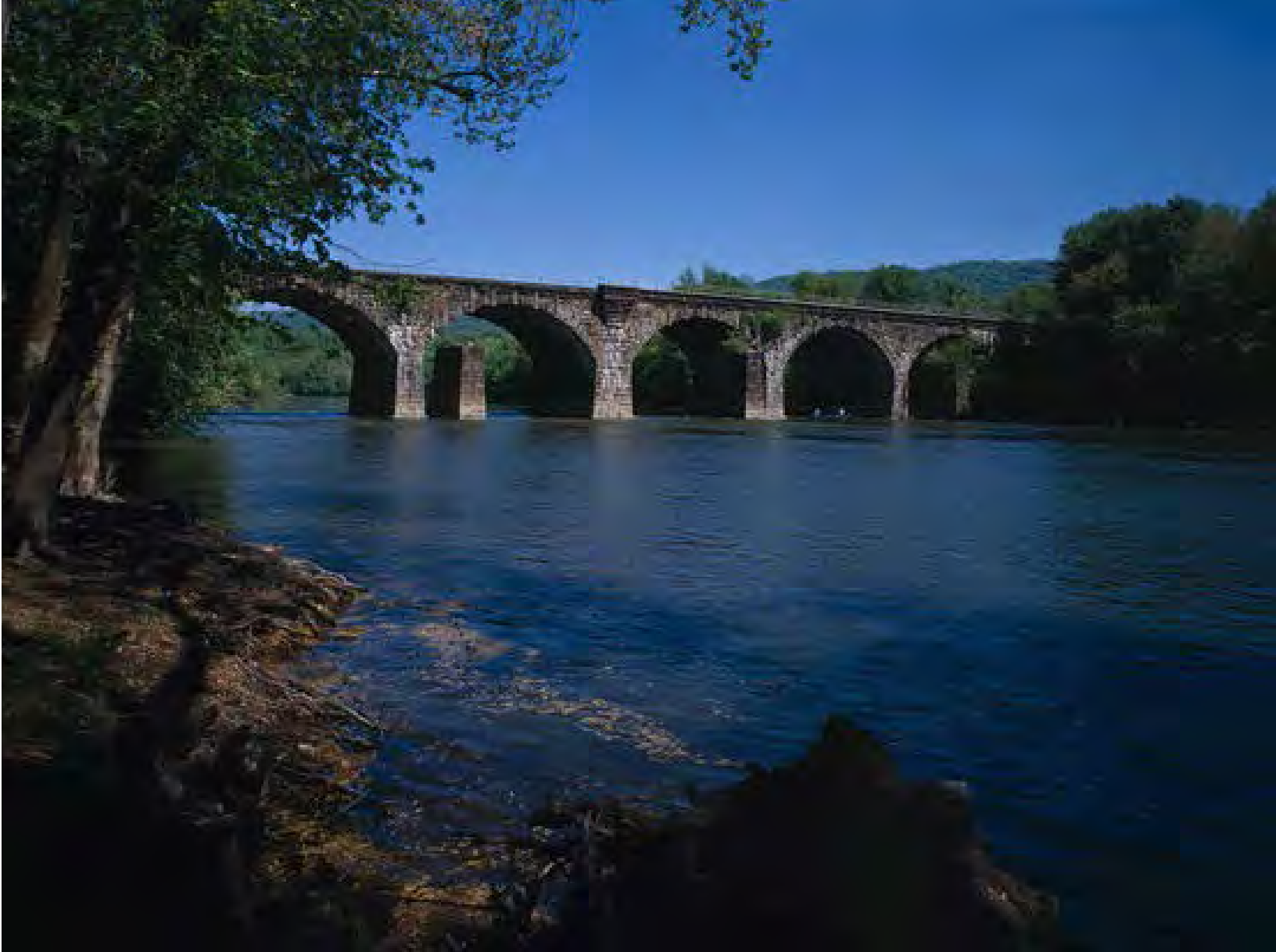
Bridge over the Juniata River, near Lewistown, PA
