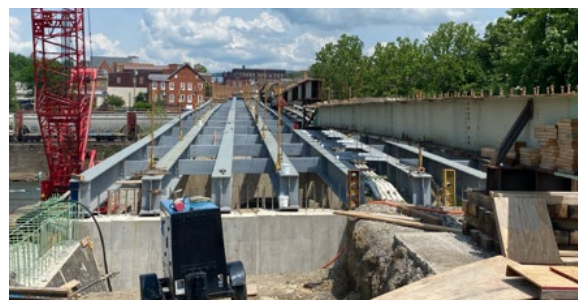
In June 2024, the new girders were placed. Photo: PennDOT District 12
