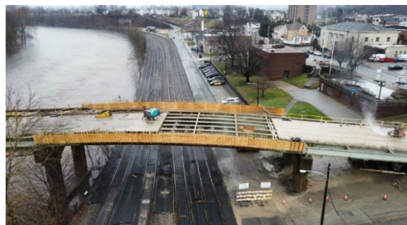
In February 2024, the demolition of the old bridge began. Photo: PennDOT District 12
