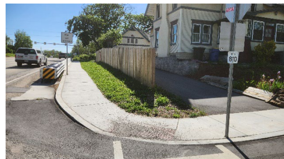
Newly constructed sidewalk with barrier along Cumberland Blvd. near 24 th St, looking east. Driveway was lowered and landscape wall and privacy fence were added to accommodate the improvement. Photo: PennDOT Connects
