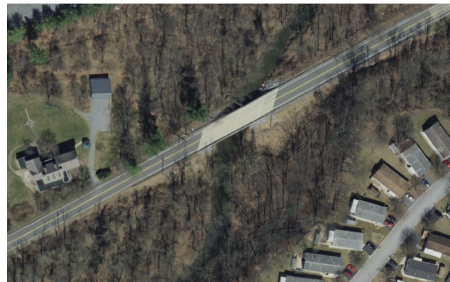
An aerial view of the new Jonestown Road bridge. Photo: PEMA
