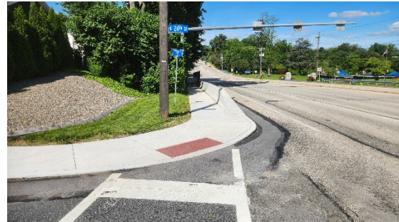
Newly constructed sidewalk with concrete barrier along Cumberland Blvd. near 24 th St, looking west. Photo: PennDOT Connects
