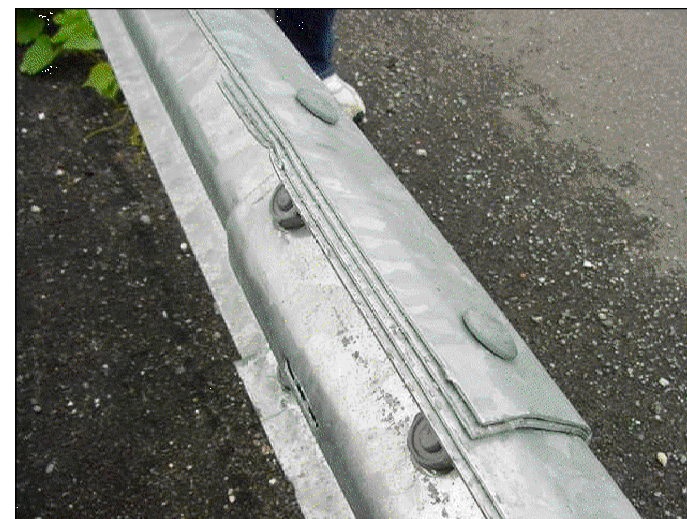
TYPICAL NESTED PANEL MID-SPAN SPLICE
