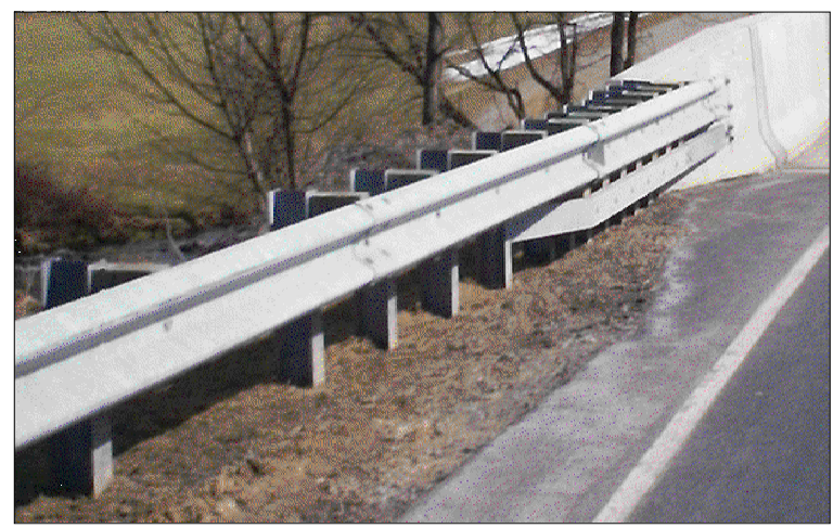
GUIDE RAIL TO TYPICAL CONCRETE BRIDGE BARRIER TRANSITION ( WITHOUT INLET PLACEMENT ) FOR DETAILS, SEE SHEET 1
