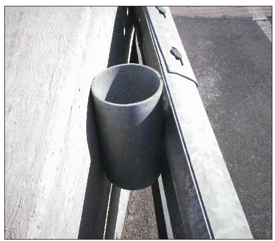
TYPICAL STEEL SPACER TUBE INSTALLATION FOR DETAILS, SEE SHEETS 1 AND 2
