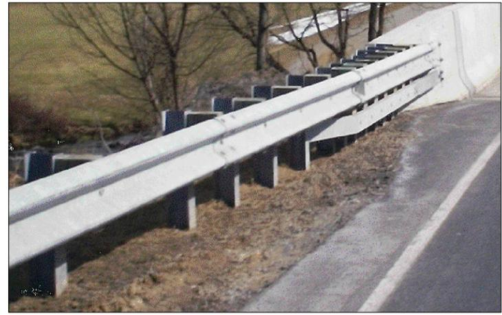
**GUIDE RAIL TO TYPICAL CONCRETE BRIDGE BARRIER TRANSITION**
