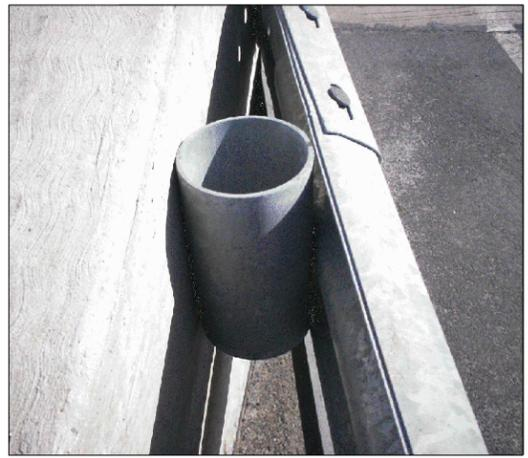
**TYPICAL STEEL SPACER TUBE INSTALLATION**
