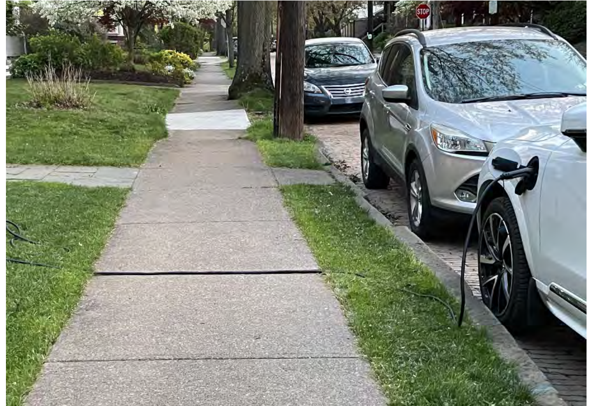
Image: An electric vehicle charging cord lays across a PA residential sidewalk without a cover. The cord must be covered to comply with federal accessibility regulations and to ensure sidewalk safety for all users.
