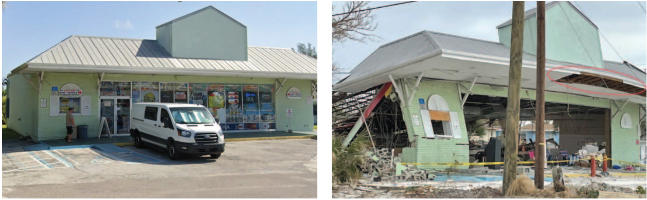
Figure 2: Example Unelevated Structure Destroyed by Flood Impact from Hurricane Ian (Source: Cotality)
