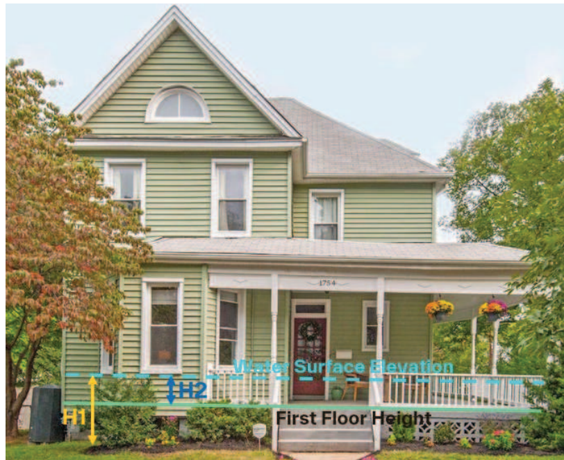
Figure 9: Concept Charts for Inside vs. Outside Tape Measurements (Source: Cotality)
