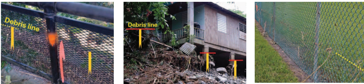
Figure 16: Debris Snag Examples (Source: USGS)
