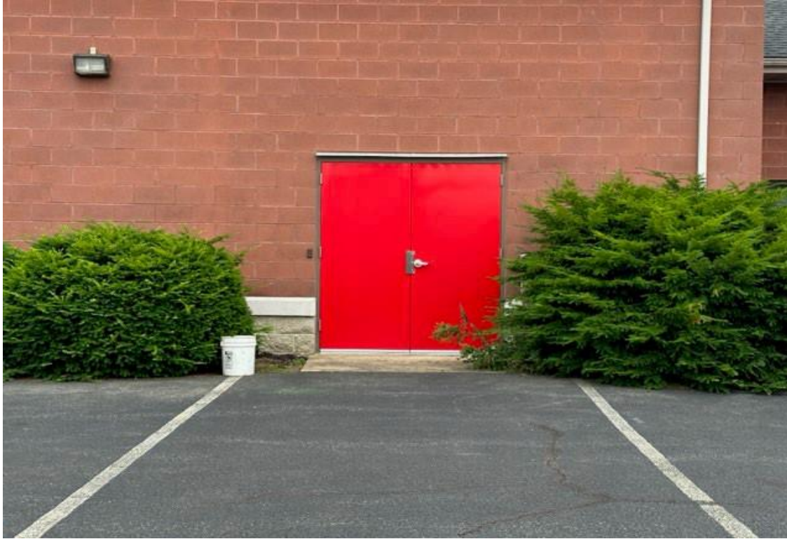
Exit Door North Side
