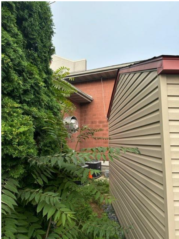
East Side Shed & Vent
