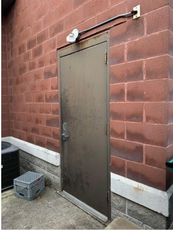
East Side Means of Exit Door
