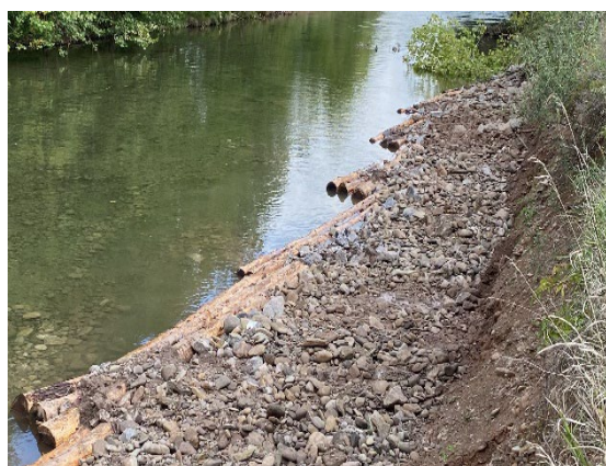
Construction of a sawtooth modified mudsill waiting for bank grading
