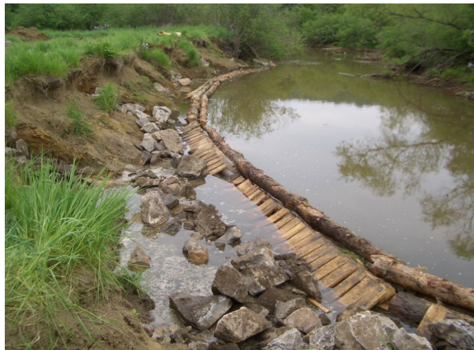
Construction of a bank cover waiting for stone and bank grading
