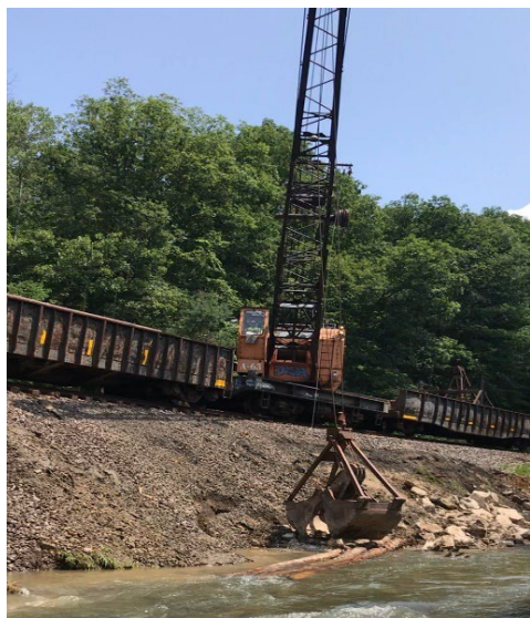
Train car crane building habitat structures
