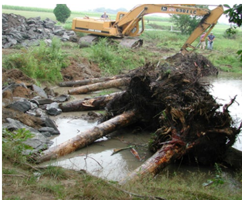
Root wads to restore lost stream bank
