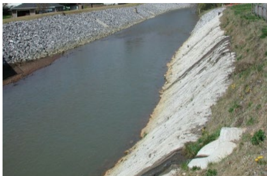
Hard surface concrete and rip-rap
