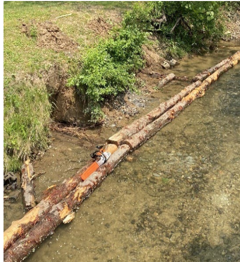
During construction of a modified mud sill
