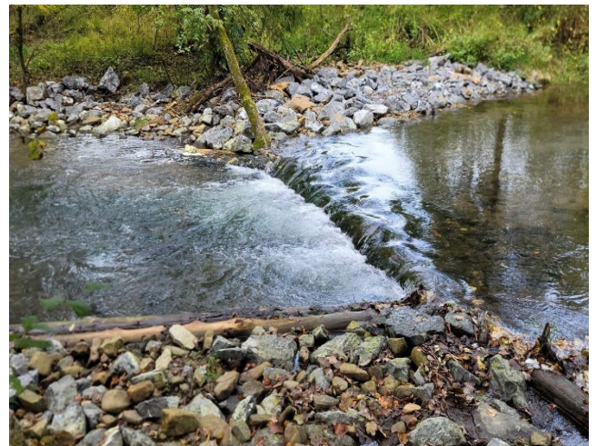
Log framed cross vane using existing fallen tree
