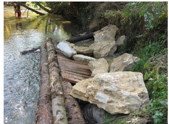
Log framed deflector using oak boards
