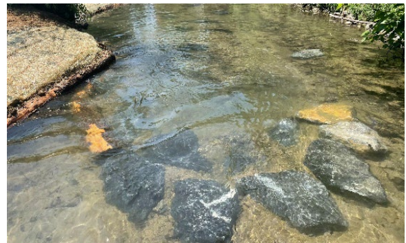
J-hook off the tip of a log framed deflector
