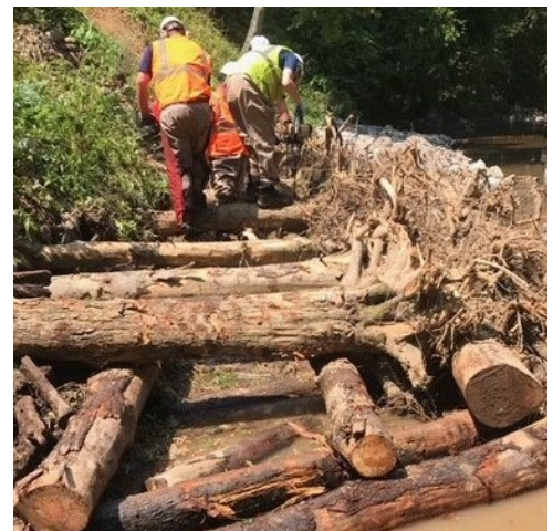
Root wad bench with cross logs to stabilize a 30-foot-high vertical cliff
