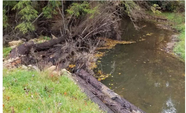
Root wad framed channel block connected to a modified mud sill
