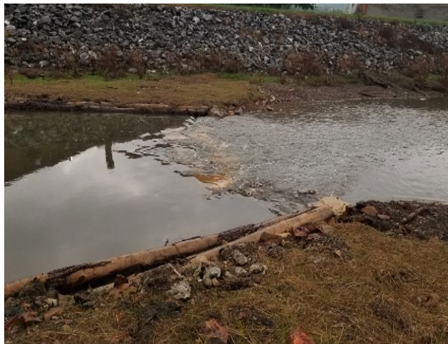
Log cross vane with rock throat
