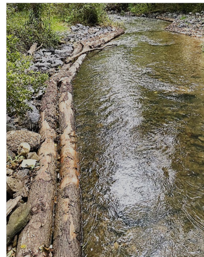
Completed modified mud sill
