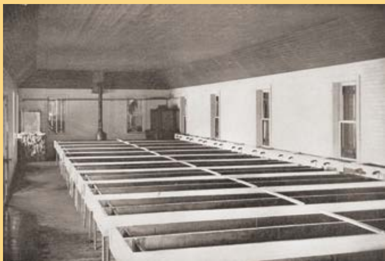
The interior of the hatchery building at Western State Fish Hatchery.
