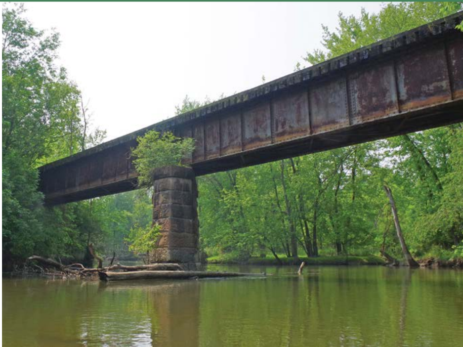
An old railroad bridge over the Shenango River, Mercer County.
