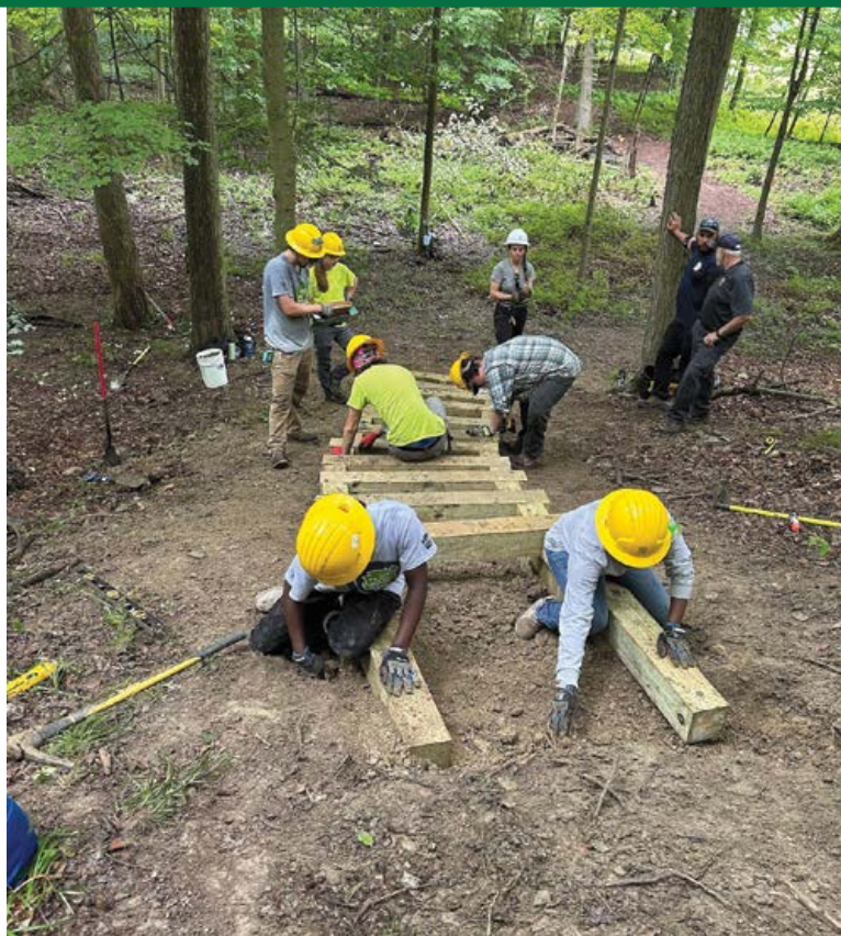
The crew placing the stairs.
