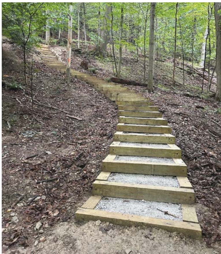
The completed stairs.
