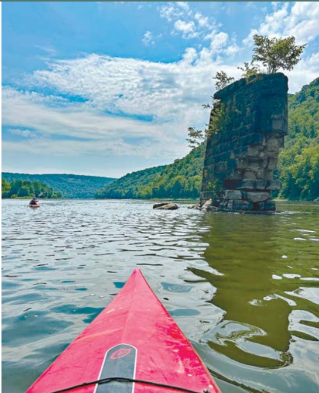
An old bridge pillar on the Allegheny River downstream of Franklin, Venango County.
