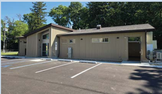
The new Lake Erie Research Unit in Fairview, Erie County.
