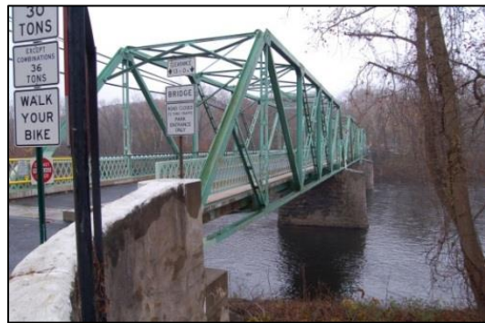
Glendon Hill Road Bridge
