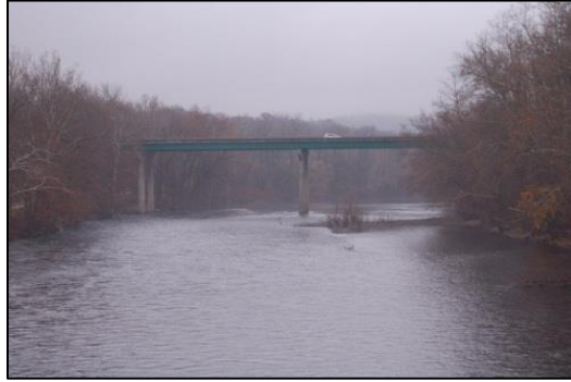
Glendon-Wilson Bridge (25 th Street / S.R. 2012)
