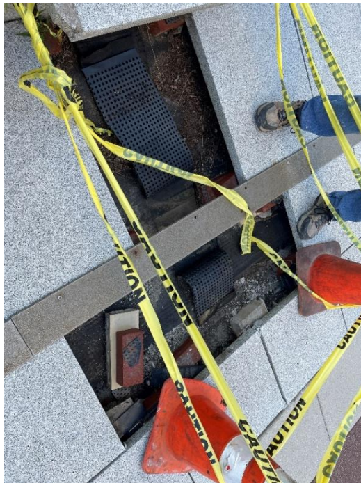
08 Probe #8 – The expansion joint cover was removed.
