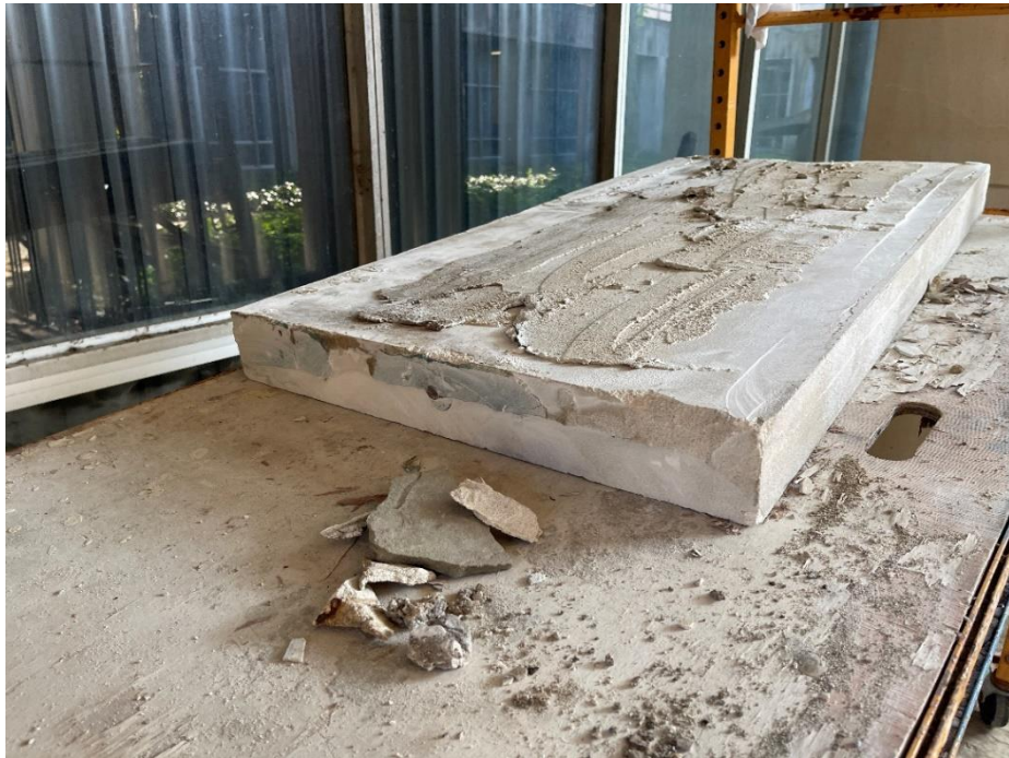
04 Probe #2 – The column facing stone was removed to observe the connection details.
