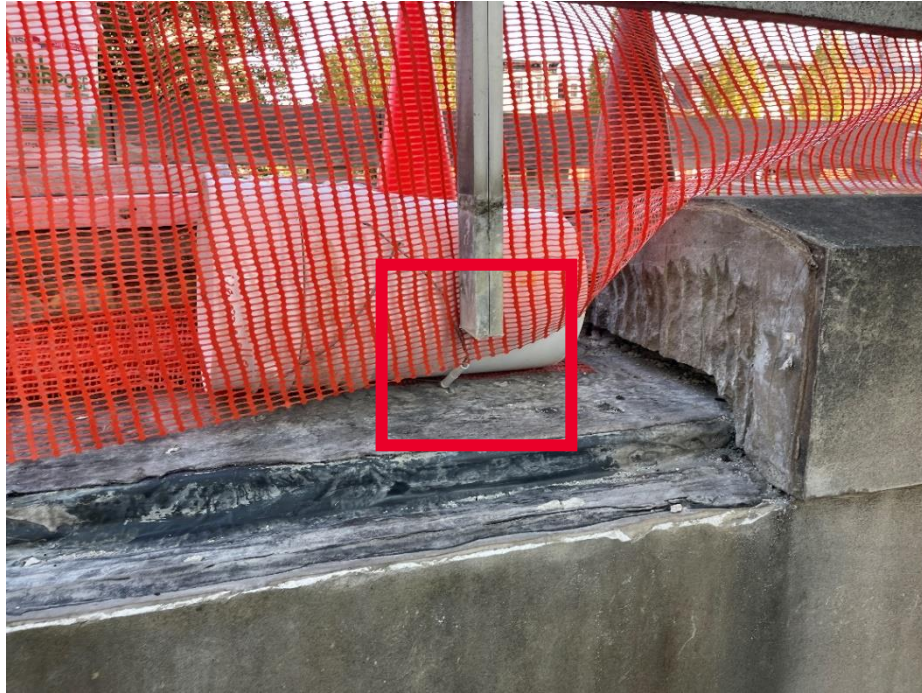
07 Probe #5 – The railing is not connected to the structural slab.
