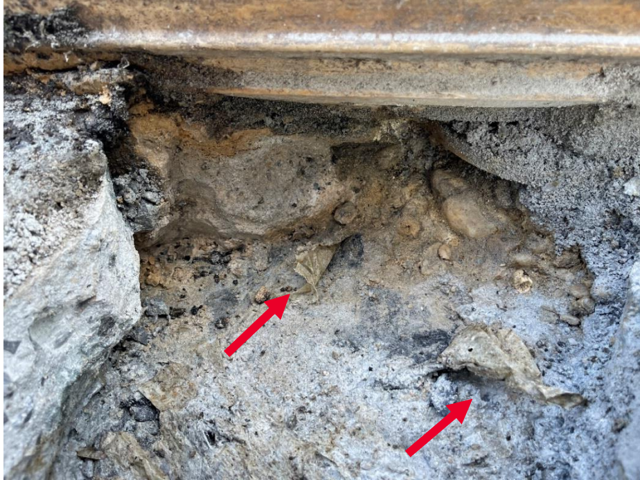
03 Probe #1 – Close-up view of waterproofing membrane.
