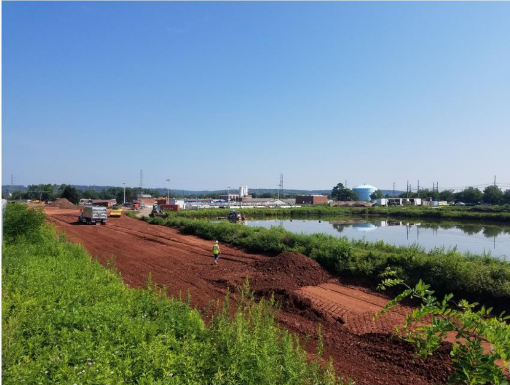
Western Drying Bed (Photo Taken from top of existing Levee near STA 703+00, looking North)
