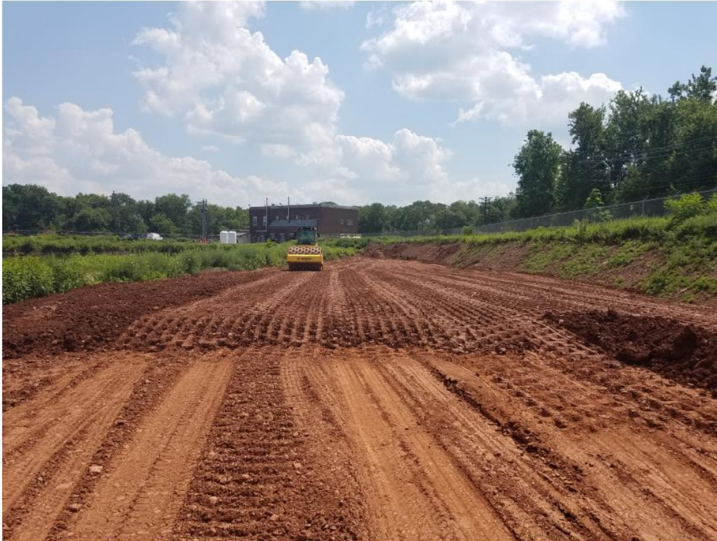
Western Drying Bed (Showing STA 705+00 to STA 703+00)
