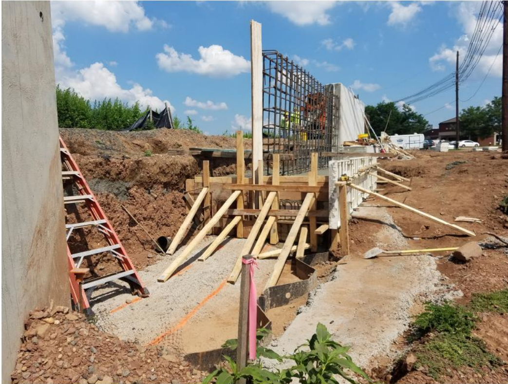
Footing poured for Monolith SE-8
