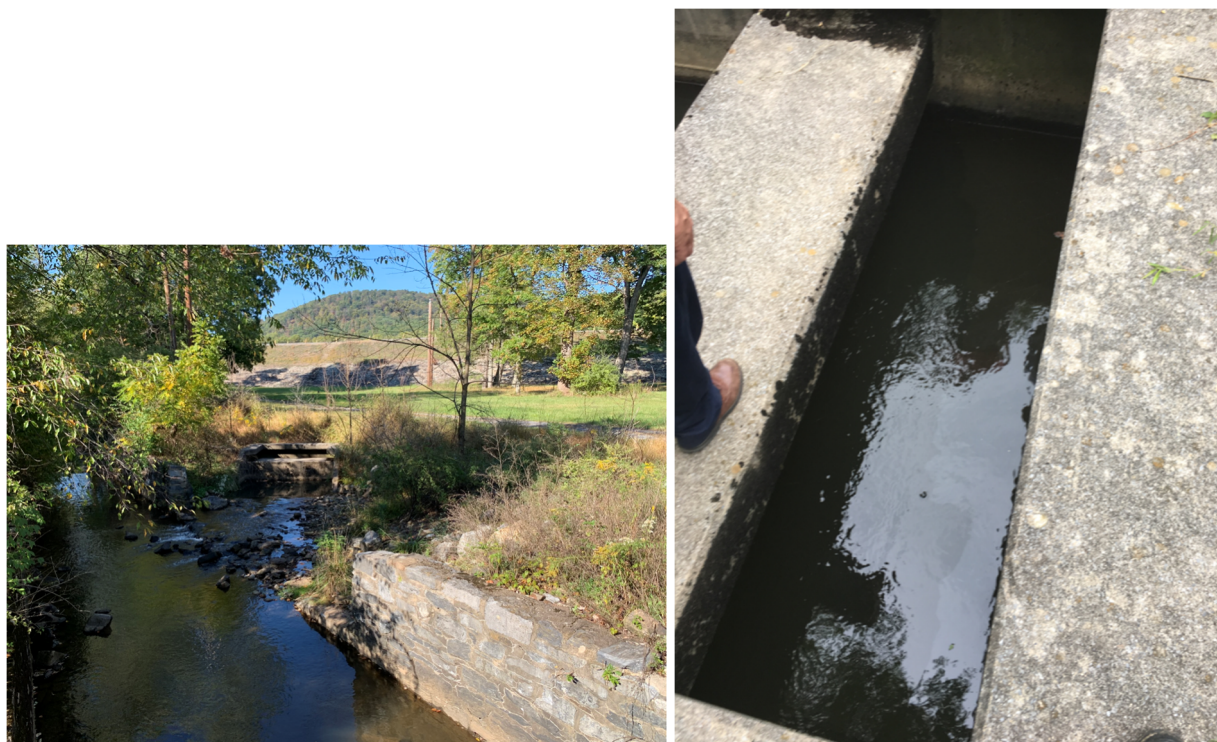
Figure 4-1– Photographs of Low-Level Outlet Works Discharge Conduit Outlet
