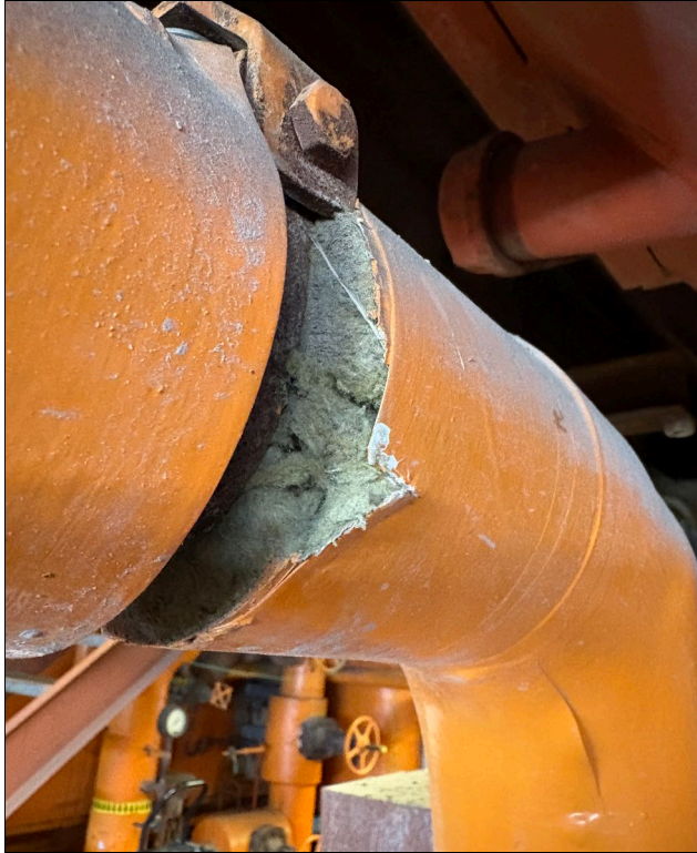
Photo 1 - HC-01A and HC-01B: White Paper Pipe Wrap and Brown Insulation
