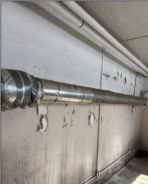
Photo 7 - HC-07: White Pipe Insulation – TSI (ACM)
