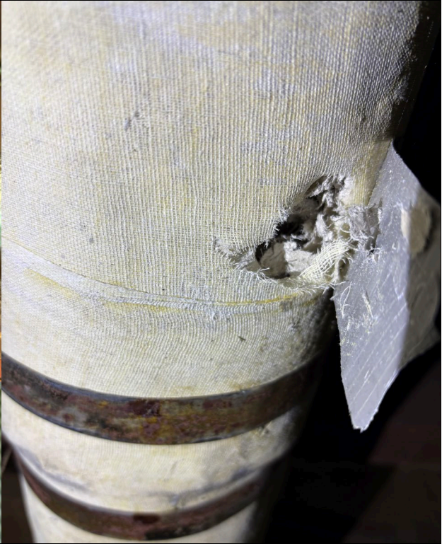
Photo 14 - HC-16: White Pipe Wrap – TSI (ACM)
