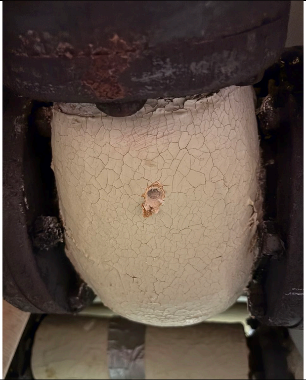
Photo 6 - HC-06: White Mudded Fitting (ACM)
