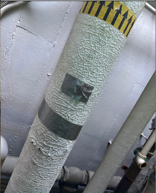
Photo 16 - HC-18: White Pipe Wrap – TSI (ACM)
