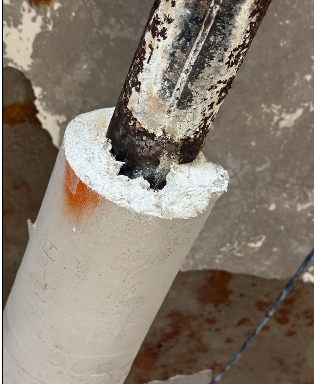
Photo 17 - HC-19: White Pipe Wrap – TSI (ACM)
