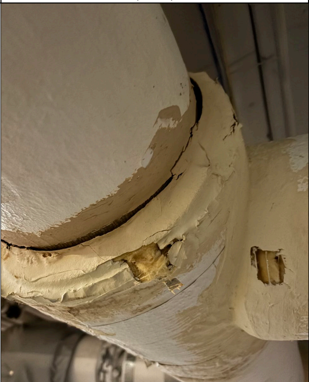
Photo 12 - HC-12 and HC-13: Tan Pipe Seam Sealant
