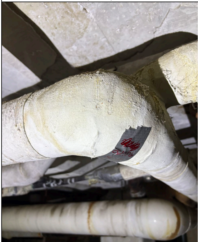
Photo 11 - HC-11: White Mudded Fitting (ACM)
