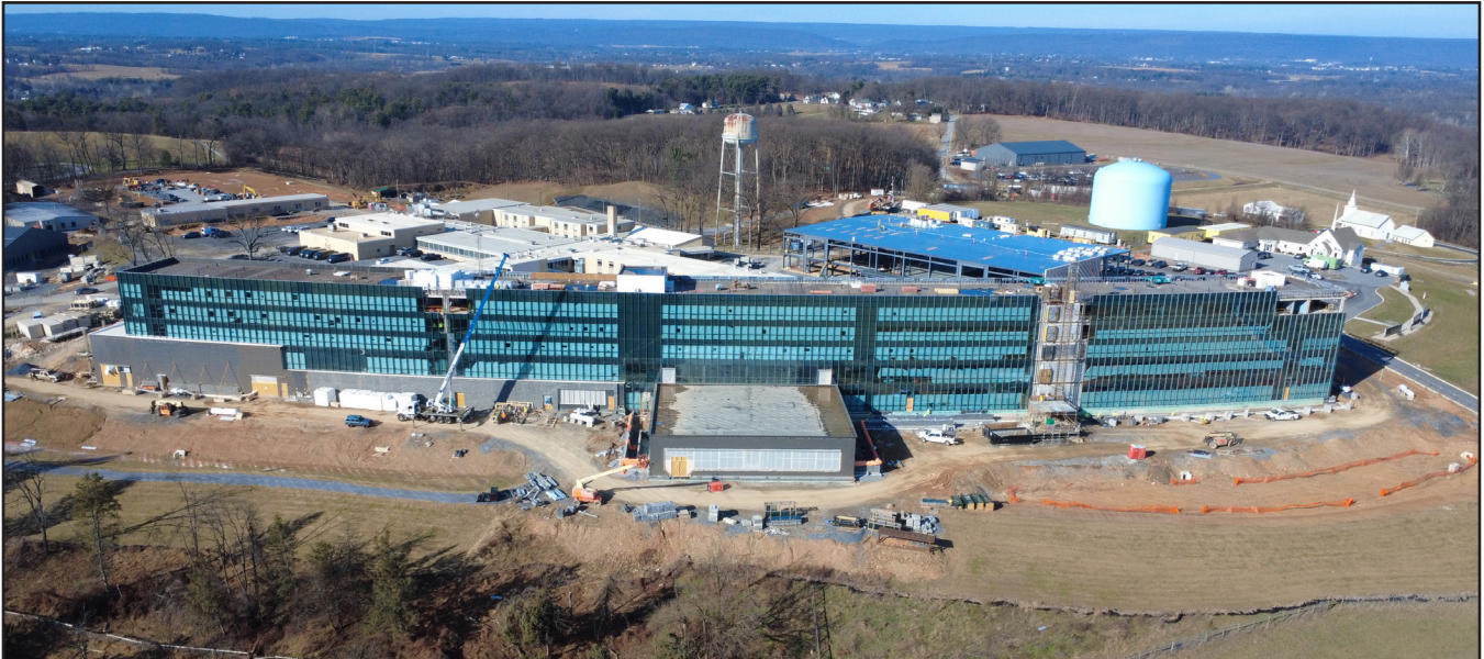
Curtainwall installation at the Marquee Building on the 147-acre active campus
