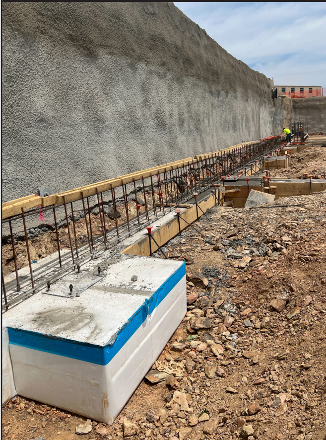
Soil wall stabilization for a deep excavation at the Marquee Building
