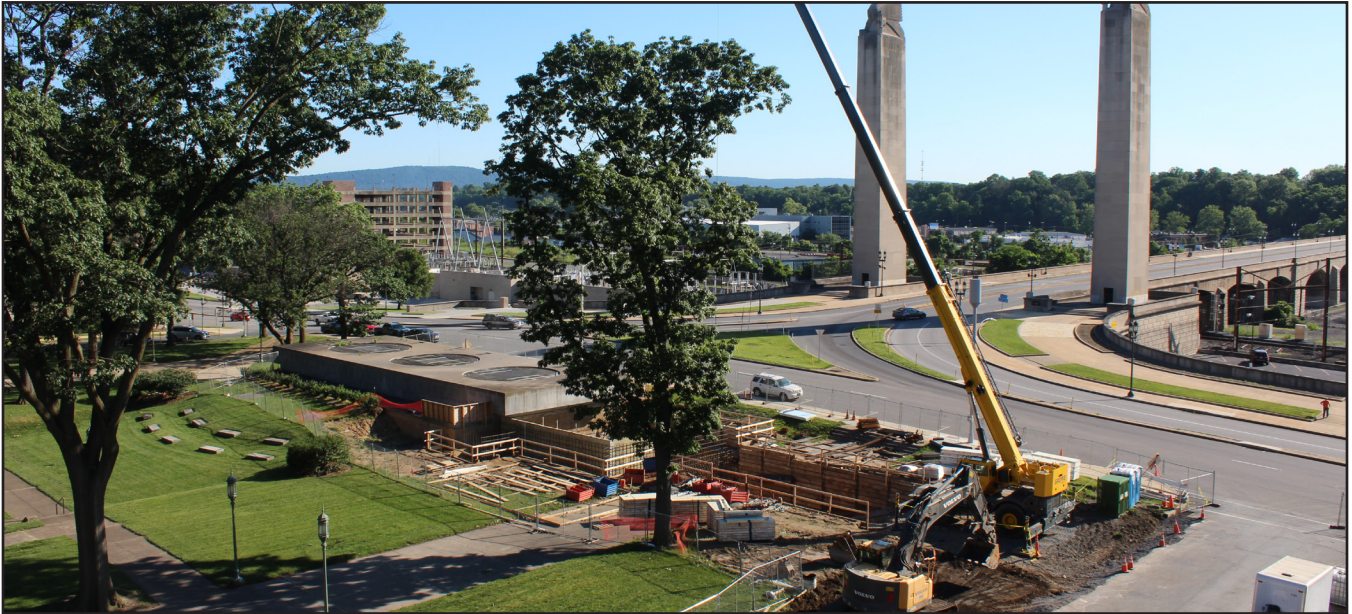
Overall completed shoring at the cooling tower expansion
