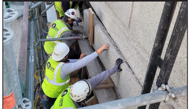
Replacing historic granite stone on exterior.
