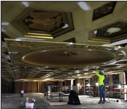
Dance floor scaffolding in place for ceiling restoration.
