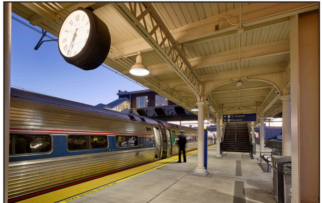
Completed historic canopy restoration.
