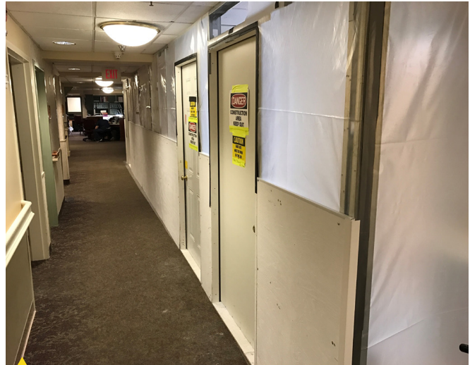
This is an example of a temporary barrier used on a recent renovation project to separate construction activities from a public space.
