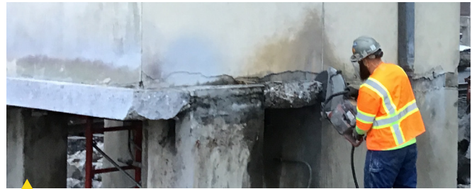
Wohlsen will implement a comprehensive silica control program in accordance with OSHA standards, including the use of wet cutting methods
