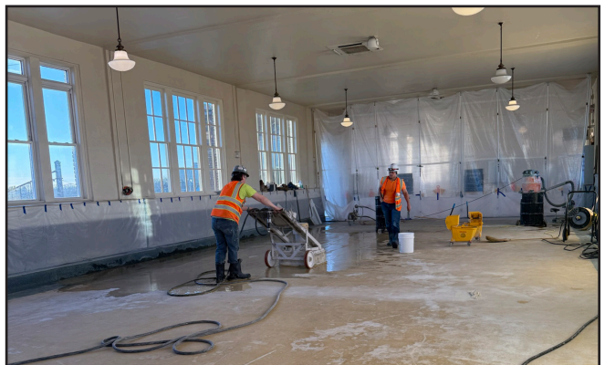
Interior renovations with floor and window restoration or replacement.
