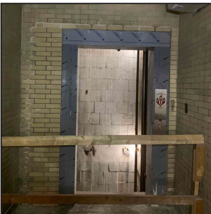
New elevator door in existing shaft.
