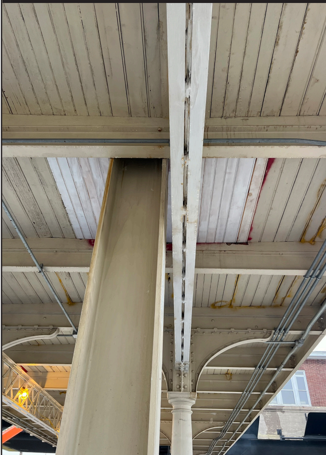
In-progress historic wooden canopy restoration.
