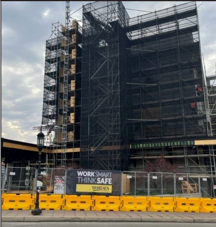
Extensive scaffolding for facade restoration showing netting and barriers for public safety.
