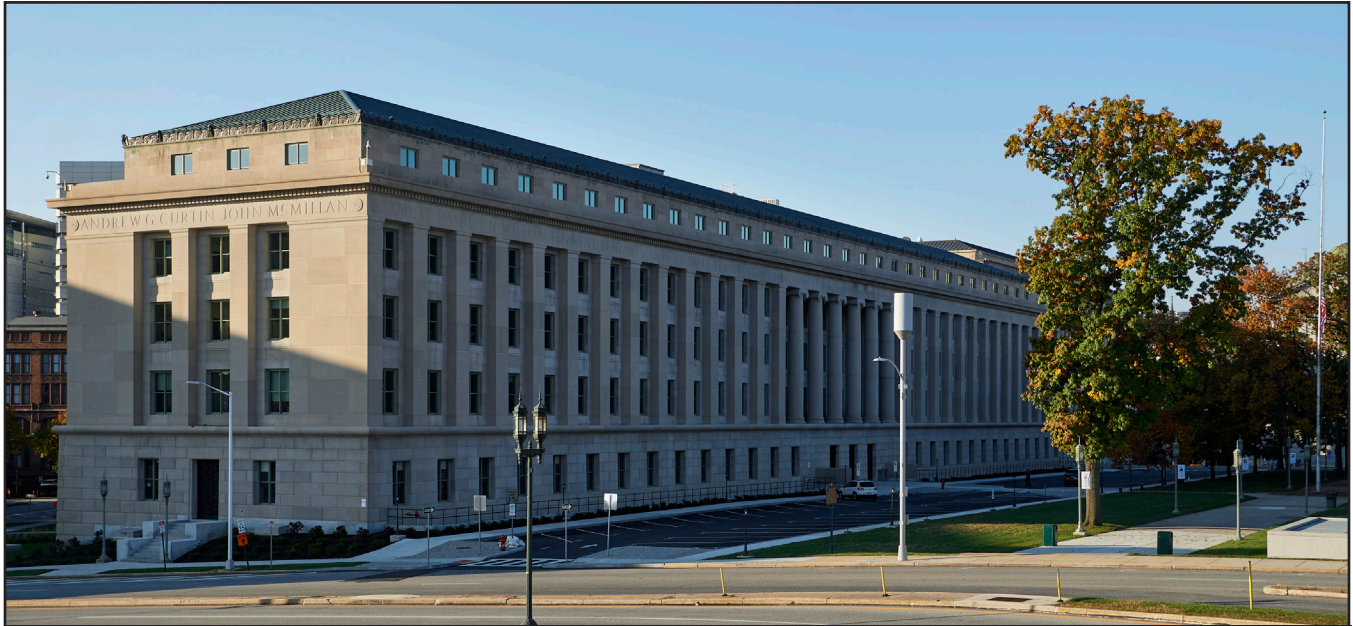
Fully restored and cleaned exterior stone and windows.
