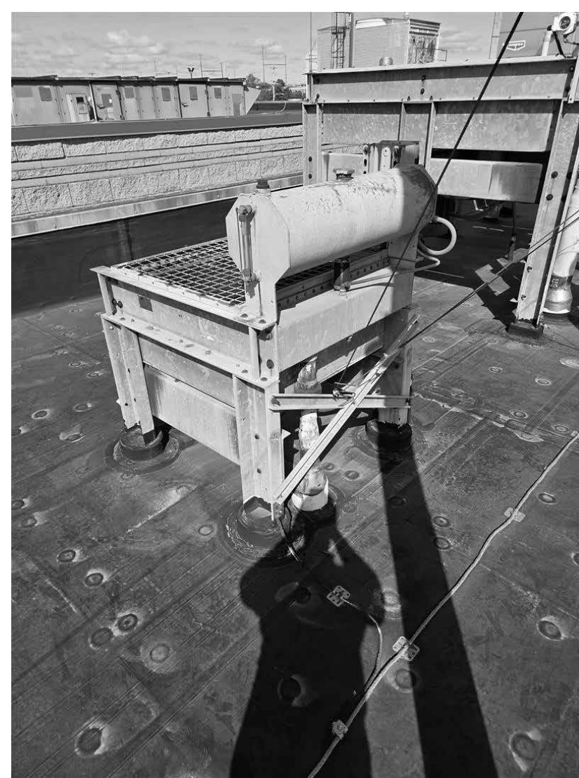
3 EXISTING GENERATOR REMOTE RADIATOR NOT TO SCALE
