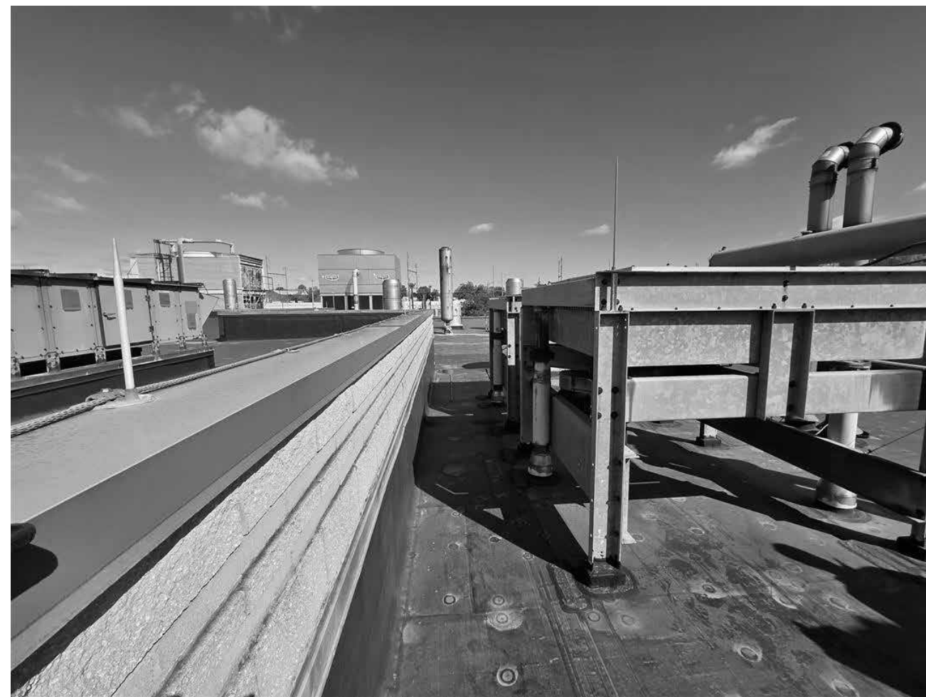
4 EXISTING GENERATOR REMOTE RADIATORS NOT TO SCALE
