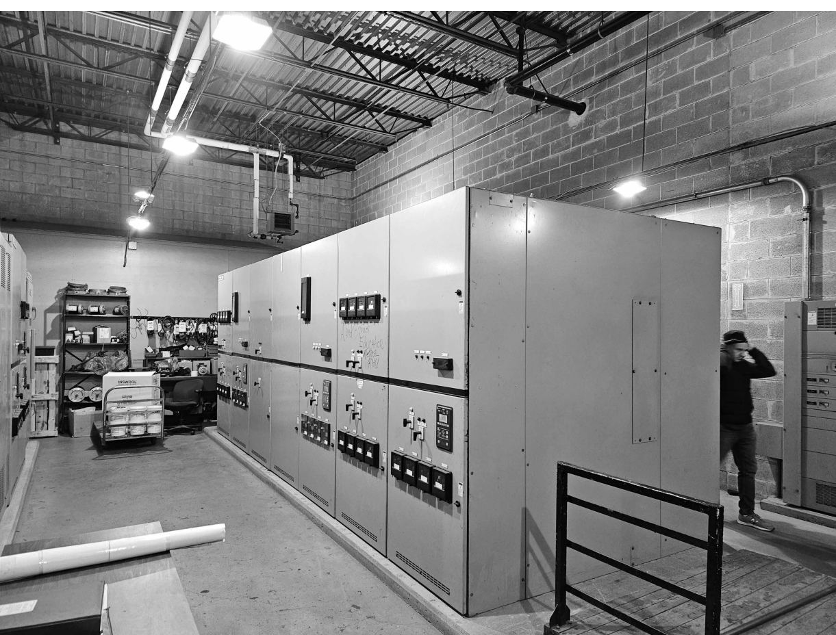
4 EXISTING MAIN SWITCHGEAR NOT TO SCALE
