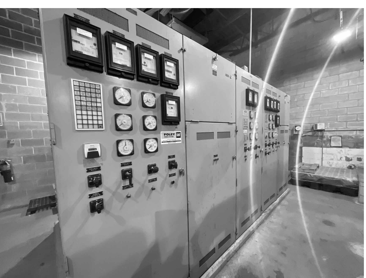
6 EXISTING PARALLELING GEAR NOT TO SCALE
